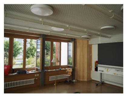
The picture shows the realisation in the classroom: The air is extracted from the room through perforated pipes suspended from the ceiling, fed into a collection duct (above the wall panel) to the 'technology cabinet' (left of the wall panel). The cabinet contains a fan for extraction, after which the air is filtered and returned to the room via a duct near the floor (below, behind the blackboard).
